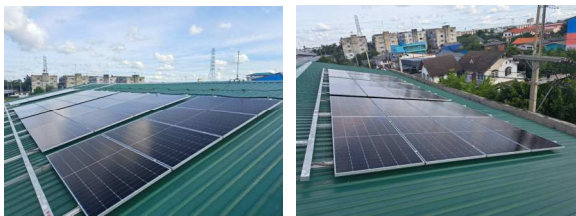
Fig. 3. Installation solar panel on the factory roof
