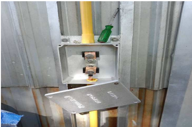
Fig. 9. Installation ground test box.
