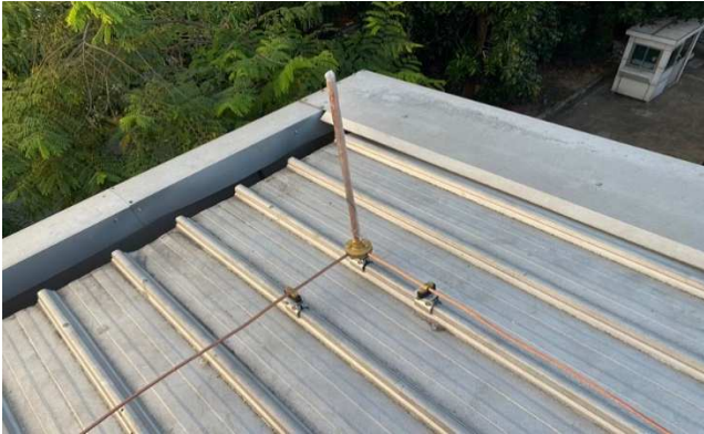
Fig. 8. Installation lightning rod.
