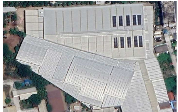
Fig. 2. Solar rooftop on the factory.
