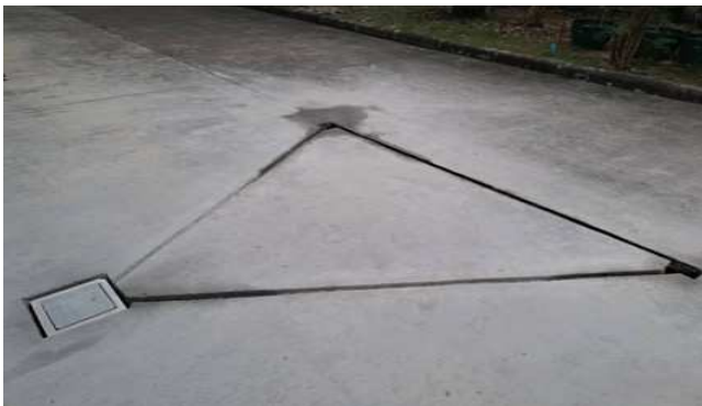
Fig. 5. Installation concrete inspection ground pit.
